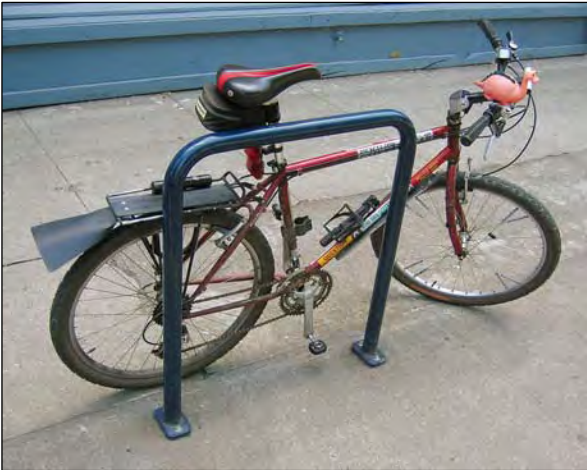
The flat top bicycle rack shown above is an example of a recommended rack type. See Appendix JJ for additional recommended bicycle rack types.
