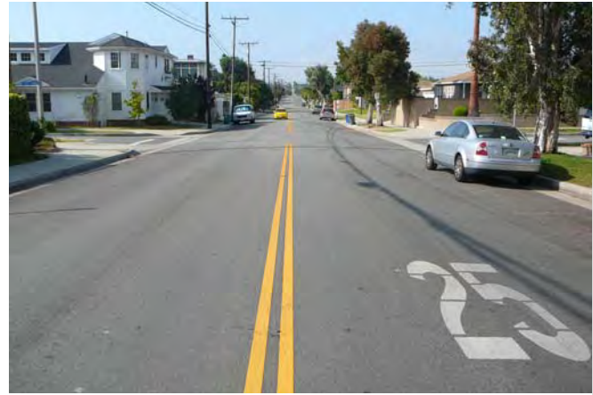
Looking south on Redondo Avenue. Pavement markings and signage will alert drivers of the presence of bicyclists
