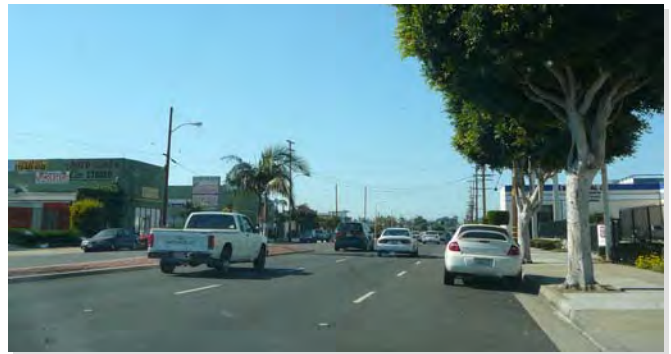
A third northbound travel lane along the center median at Rosecrans Avenue does not provide adequate roadway width for a bicycle lane.
