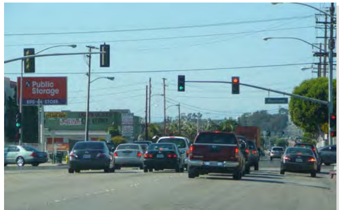
Bicycle detectors at signalized intersections will position bicyclists to trigger the signal when no vehicles are present.
