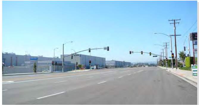
Looking south on Douglas Street. The northern portion of Douglas Street has wide lanes that could be narrowed to accommodate bicycle lanes.
