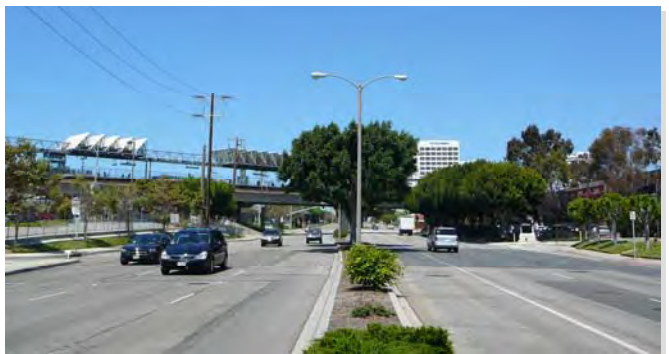
East of Sepulveda Boulevard, El Segundo Boulevard has six travel lanes and high volumes of vehicular traffic. A cycle track will provide protection for bicyclists.
